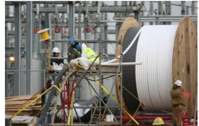
Photo courtesy of Southwire
