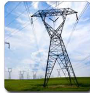
High Power Transmission Cables (AC)
