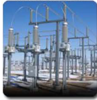
Superconducting Fault Current Limiter
