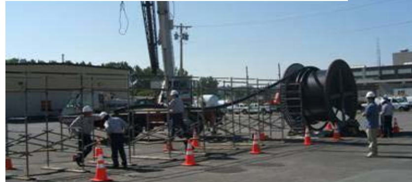
Installation at Albany Cable site (Aug. 5, 2007)
