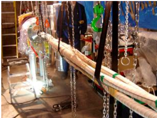
3 Cable cores after connecting
