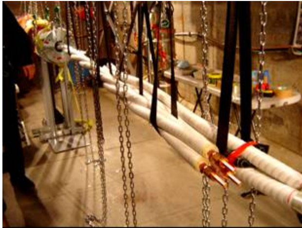
3 Cable cores before connecting
