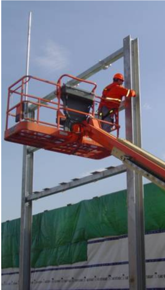
Take-Off Structure Installation
