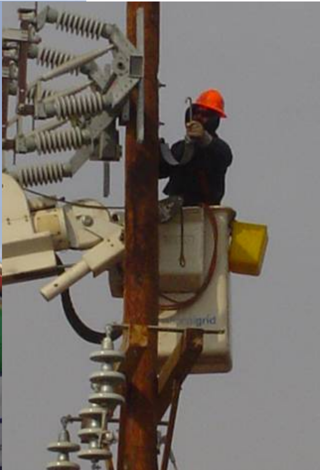
Installation of Disconnect Switches
