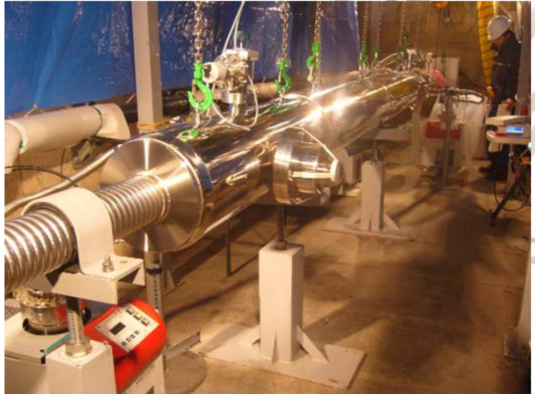
Joint box with vacuum vessel (before covering with water-tight tapes)
