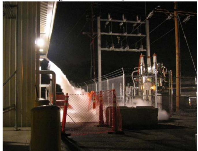
Fig. 5. Liquid nitrogen venting at end of the cooldown process.
